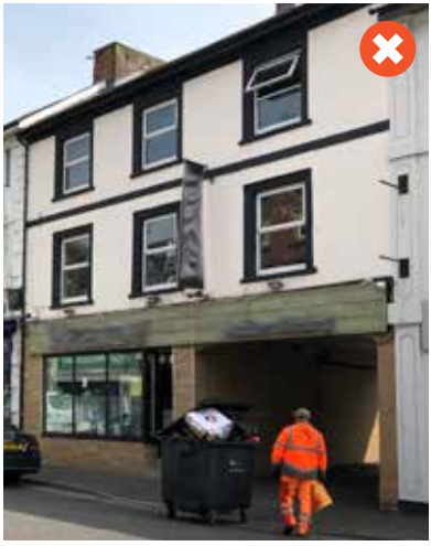
Figure 12. Fascia applied obscuring archway
