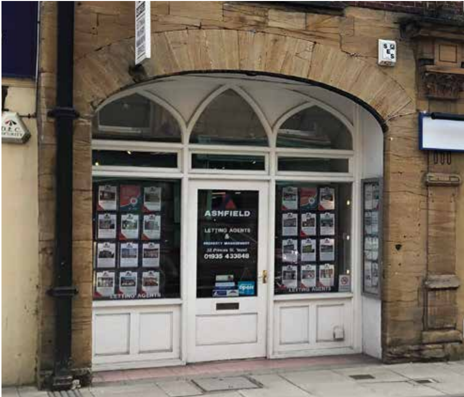
Figure 25. Recessed doorway, shopfront style matches building setting, panelled stallriser
